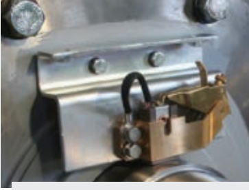
■ A shaft ground brush assembly mounted on drive end of the motor.
