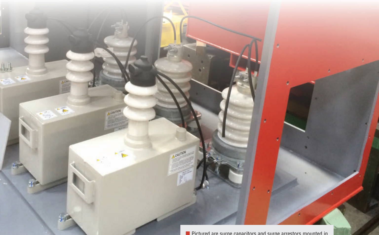
■ Pictured are surge capacitors and surge arrestors mounted in a terminal box.
